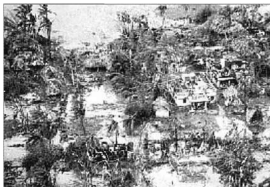
Destruction caused by a cyclone
