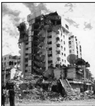
Fig. 3.3a: Destruction caused by an Earthquake in Gujarat
